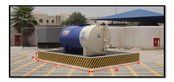
Storage Tank Bundwall should be constructed using concrete material and should be plastered inside & outside and the concrete base should be 10 centimeter thickness. Fabricated steel plate bundwall is also allowed.
