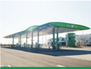
CNG Fueling Station
