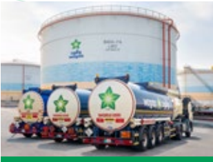
Fuel Storage and Distribution
