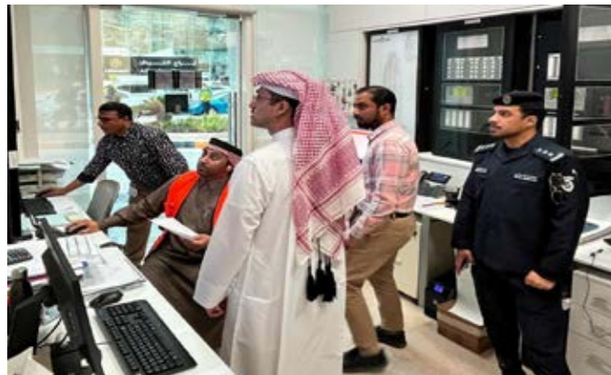
Qatar Civil Defense Officers and WOQOD monitoring the unannounced exercise at WOQOD Tower Fire Command Center
