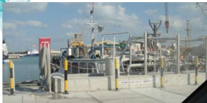
Berth expansion project (Diesel & Water Dispensing) - Ras Laffan
